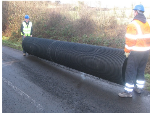
Figure 4. DN600 polyethylene steel reinforced pipe lifted by two operatives.
