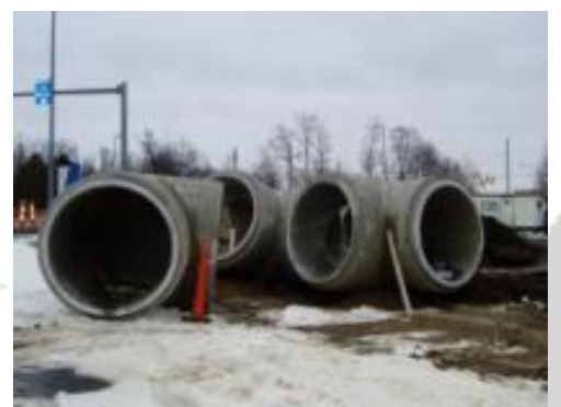
72-inch diameter bends and tees.
